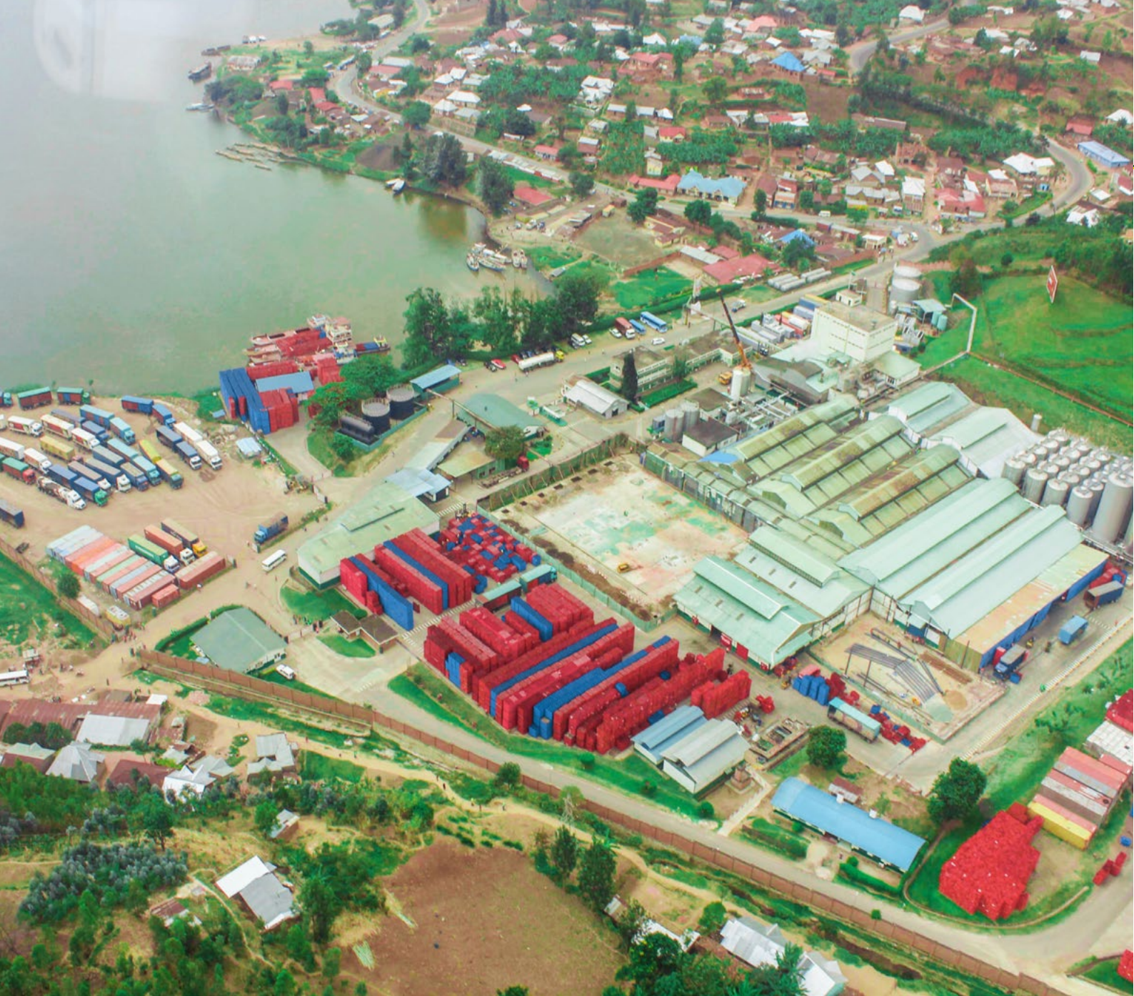
Aerial view of Gisenyi brewery site
